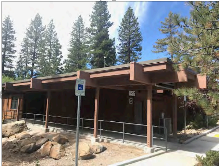
Figure 4 Incline Monitoring Station
